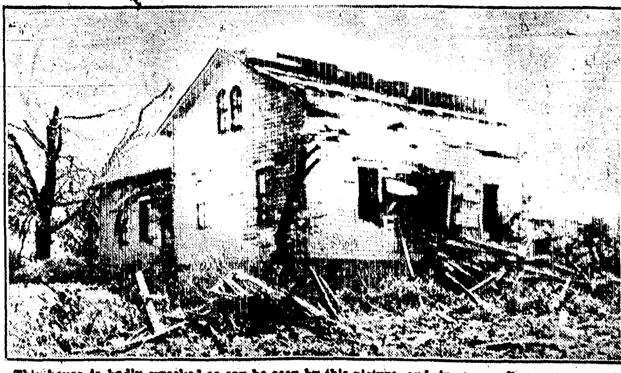
This house is badly wrecked as can be seen by this picture, and in a peculiar manner. The house belongs to A. Claude Wilson, Wheatland township, Hillsdale county, and the cyclone which struck there June 20, 1937 did this damage. This wreck was caused by flying boards and timbers from a house across and about 20 rods down the road, belonging to a neighbor, and which was totally destroyed by this windstorm. Mr. Wilson's barn was also completely destroyed besides considerable other damage was done. This company promptly paid the loss as follows: $1000 on house, $1800 on barn, $133.33 on silo, $75 on windmill, $24 on furniture, $80 on livestock, $144 on farm tools, $50 on hay and grain and $125 other damage. It paid this policy holder to have windstorm insurance with this old company.
